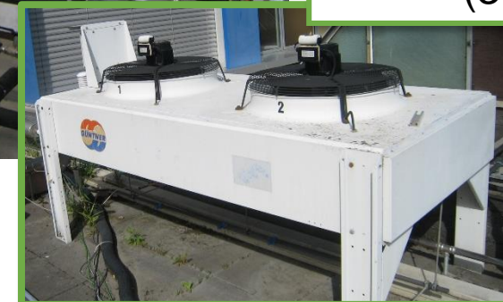
Emulation of space heating loop (30kW)
